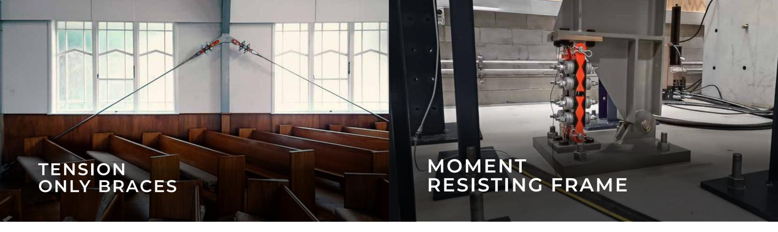
The Tectonus devices provide the tension fuse to the braces and prevent out-of-plane buckling.
